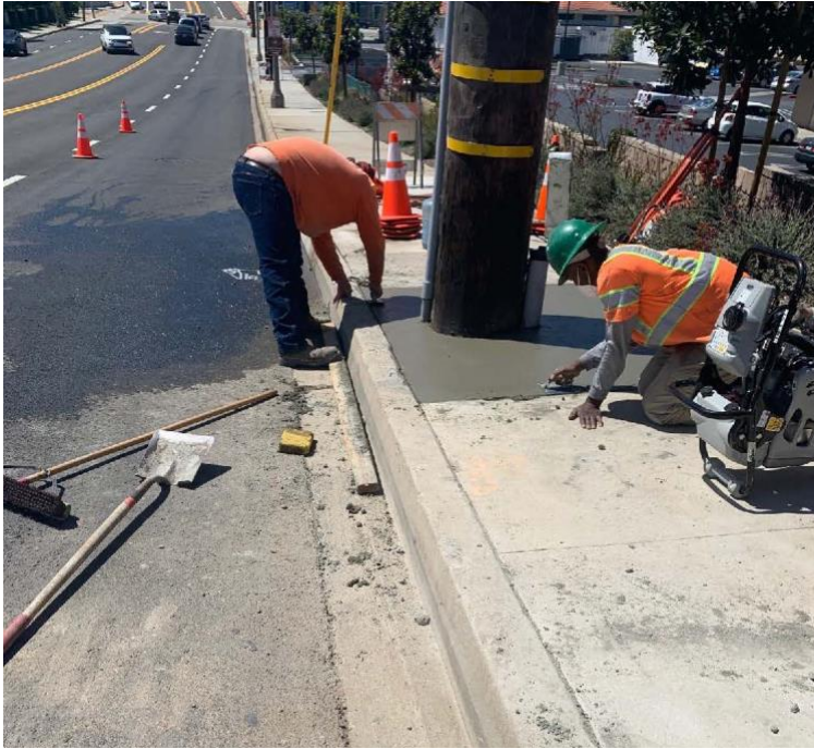
Construction crews working at SBFN connection site
